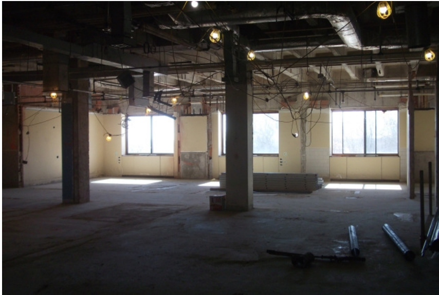
New Plumbing for 5 th Floor Above
