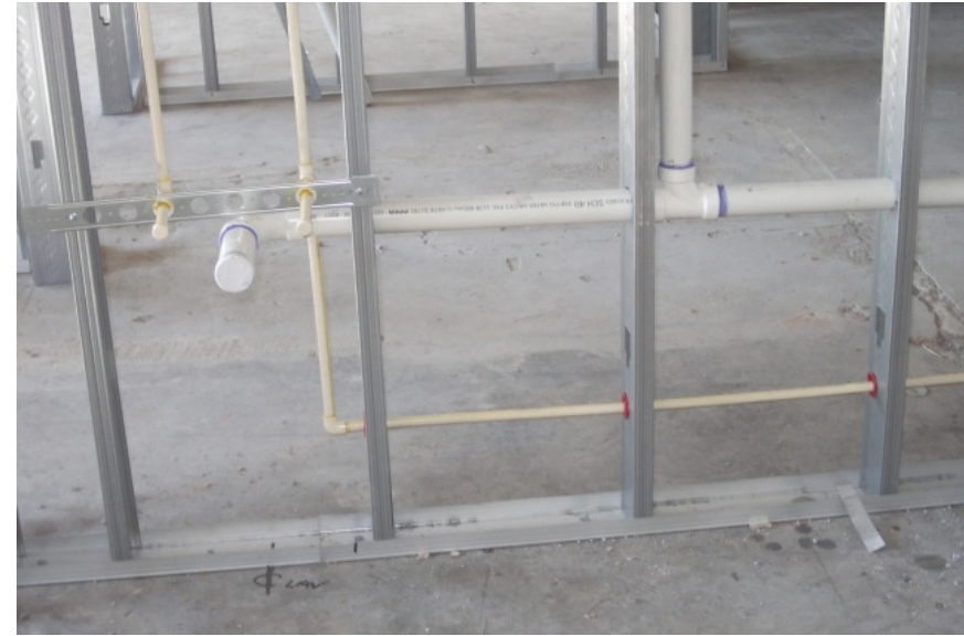
New Bath Plumbing
